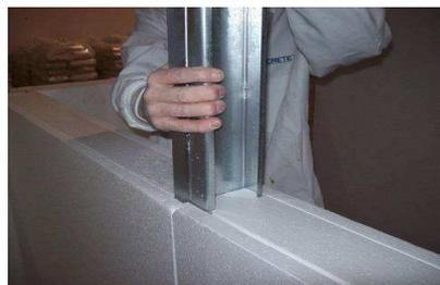
Insert studs and panel to panel inline connectors. Connectors fit into the bottom track and fit flush with the top of the panels.
